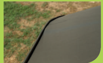
Front drain pipe diverts rainwater
